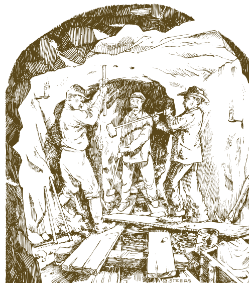
Working by candlelight, miners dug more than a half-mile of tunnels beneath Mine Hill using only hand tools and black blasting powder. The three main tunnels had rails laid inside them, with the bottom tunnel connected to the Donkey Trail for transporting the ore to the roasting ovens.
